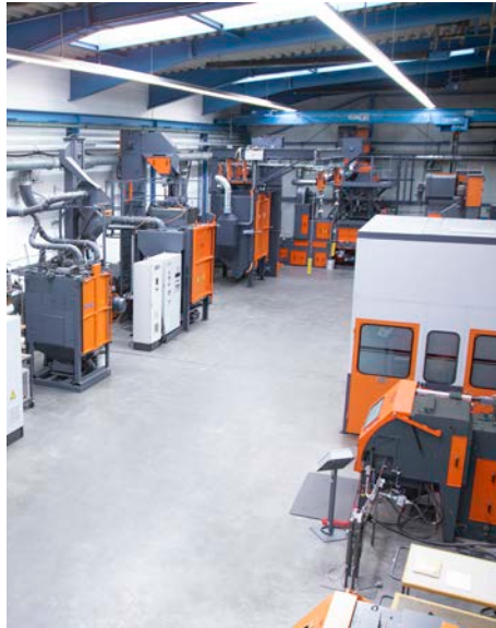
CEC Shot Blasting
